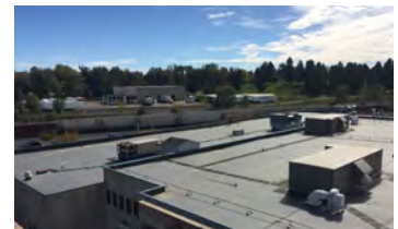
Image 2.1: Recently replaced Annex Building roof
