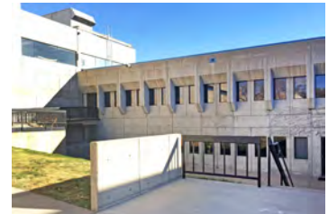
Image 2.0: West Facade - Annex Building
