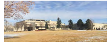
Image 1.0: Southwest Facade - Main & Annex Building
